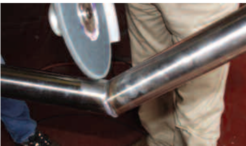
Treatment of the inside angle with an internal angle finishing tool
